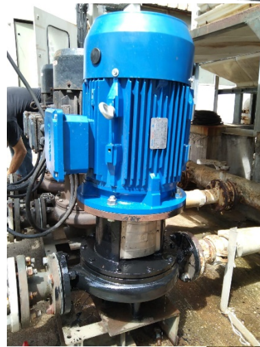
• Vertical In-line Pump
